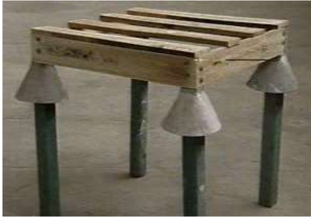
Fig. 7. Aluminium cones on pillars
