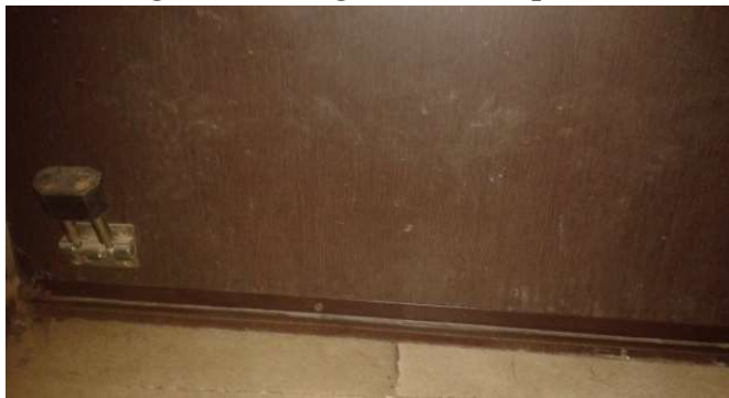
Fig. 9. Galvanized iron sheet on lower border of the door
